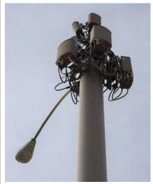
Avoid New Equipment Protruding from the Pole Avoid Exposed Wiring and Creating Obstructions
