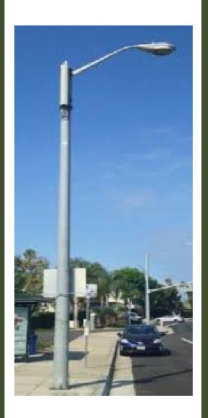
Required Aesthetic Standard for Replacement Poles or New Structures on Light Poles (luminaire placement may vary depending on existing street light installations)
