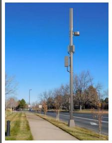
Avoid Antennas Protruding from the Pole and Avoid Incompatible Antenna Installations along the same street
