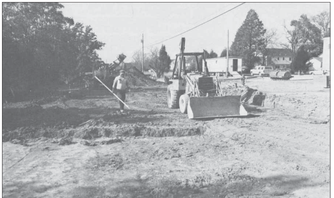
Construction on Grigsby Chapel road from the late 1980s.
