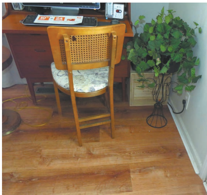
By taking up worn, wrinkled carpet and replacing with vinyl laminate flooring, a serious trip-hazard is corrected.
