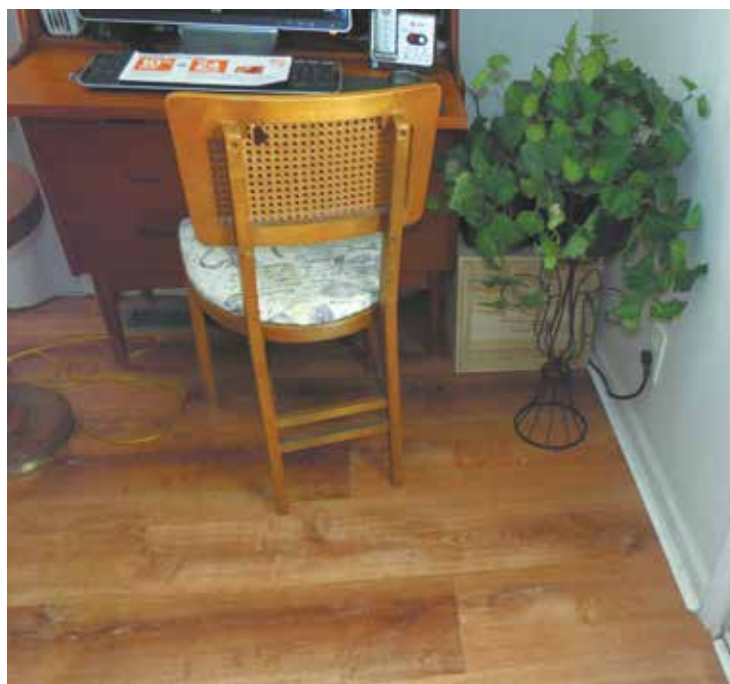
By taking up worn, wrinkled carpet and replacing with vinyl laminate flooring, a serious trip-hazard is corrected.
